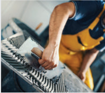
GLUING THE SLAB
