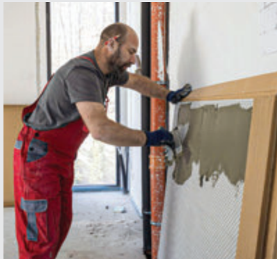
GLUING THE SLAB
