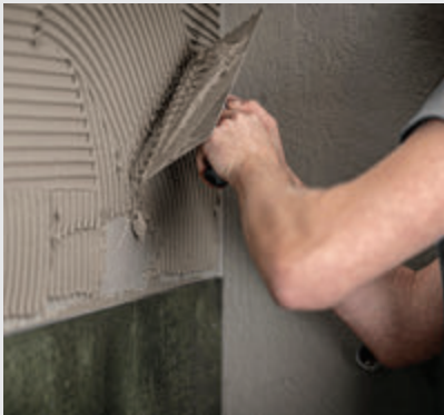
GLUING THE SUPPORT
